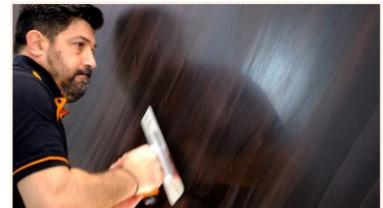
**IMPORTANT: After the polishing process, a thorough hand polishing with the stainless steel trowel is still required**
