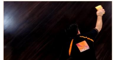
After waiting 10-15 minutes, polish the surface with a stainless steel trowel using an adequate pressure on the surface.
